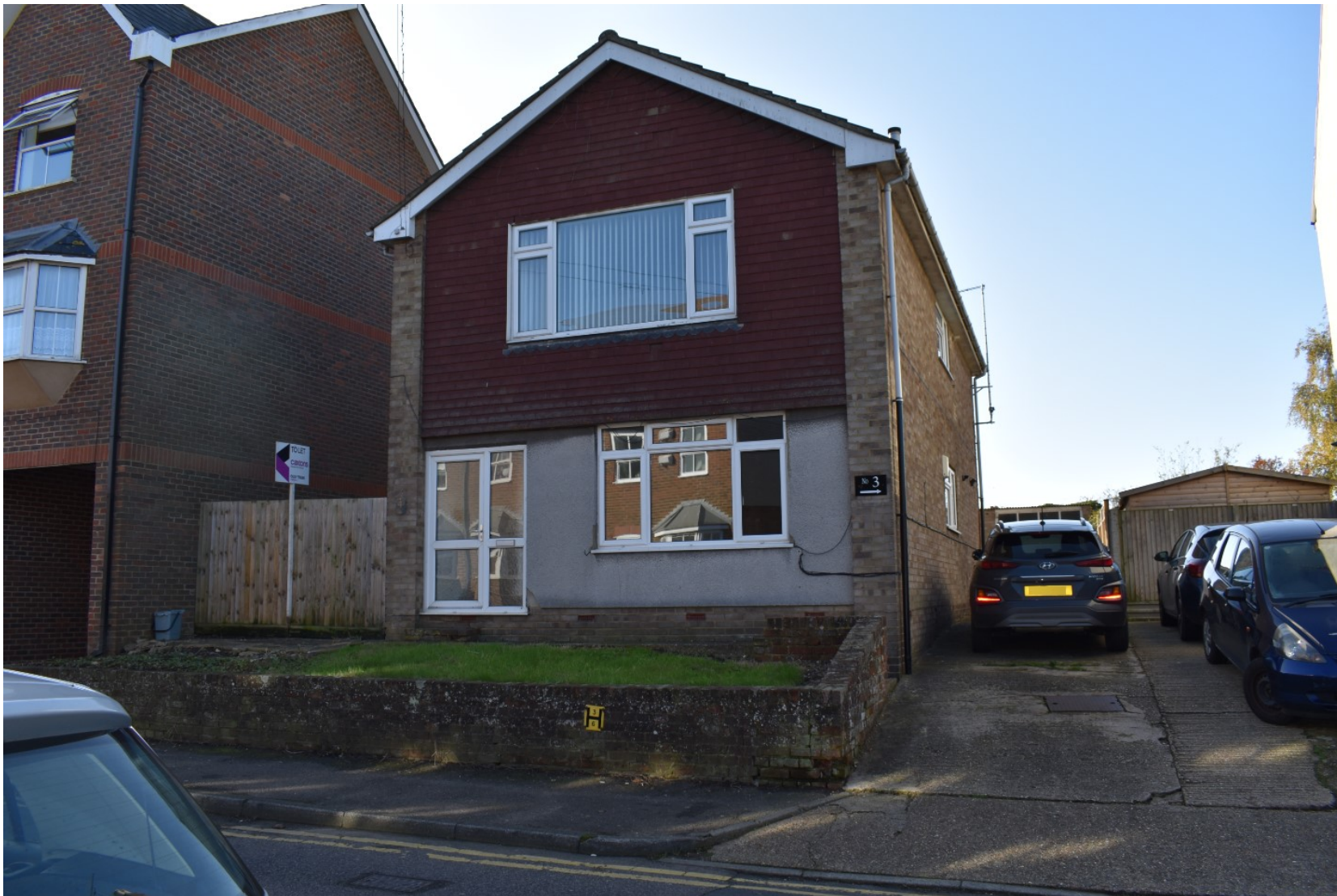
Plate 7: View of front (facing S)
